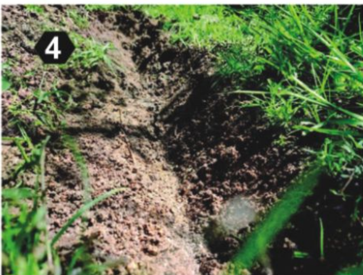
4 Dig a pit of 3-5 inches depth
